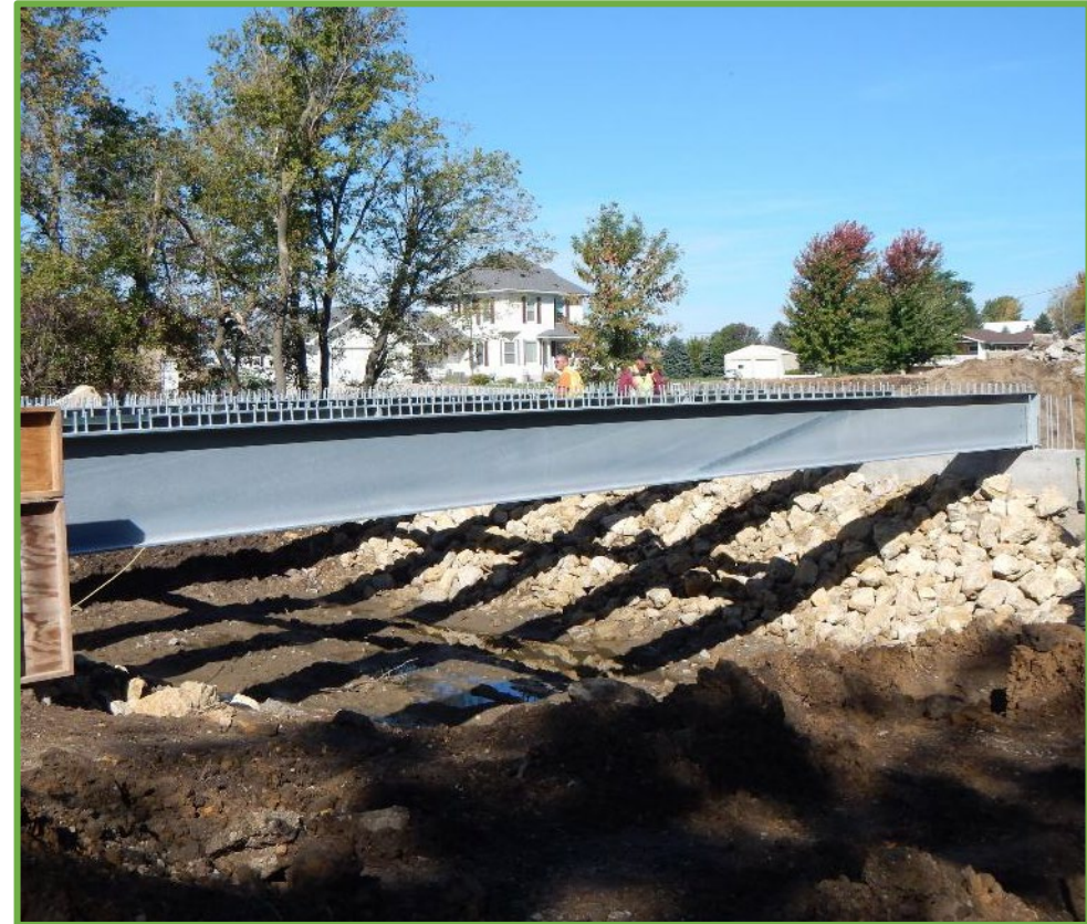
Progressive Dipping: 63 ft Bridge Girder Jesup South Bridge Buchanan County, Iowa | 2013
