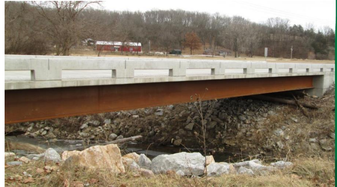
Superstructure Design for Two-Lane, 80 ft Simple Span Bridge
