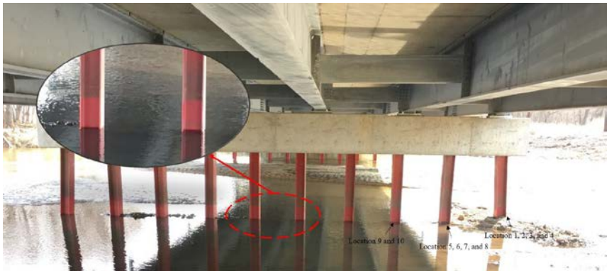
c) Galvanized and painted piles
