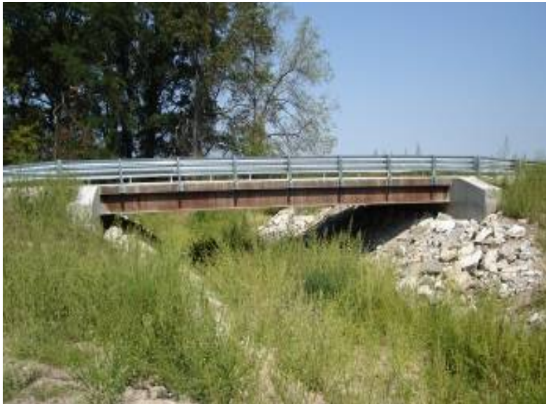
Audrain County, MO Bridge 411
