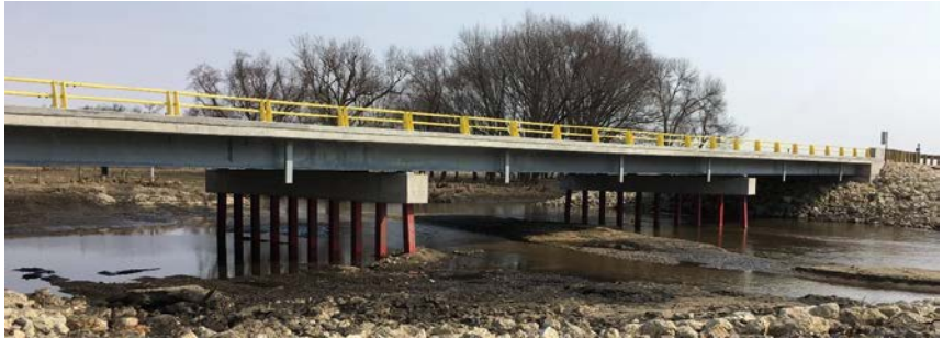
a) Bridge side view (with water level low)
