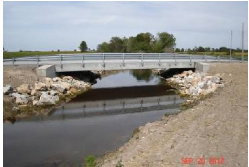
Audrain County, MO Bridge 336
