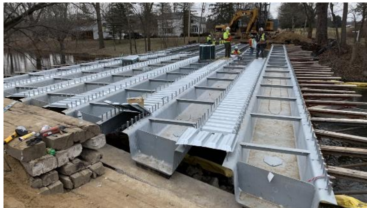
Press-Brake-Formed Tub Girders
