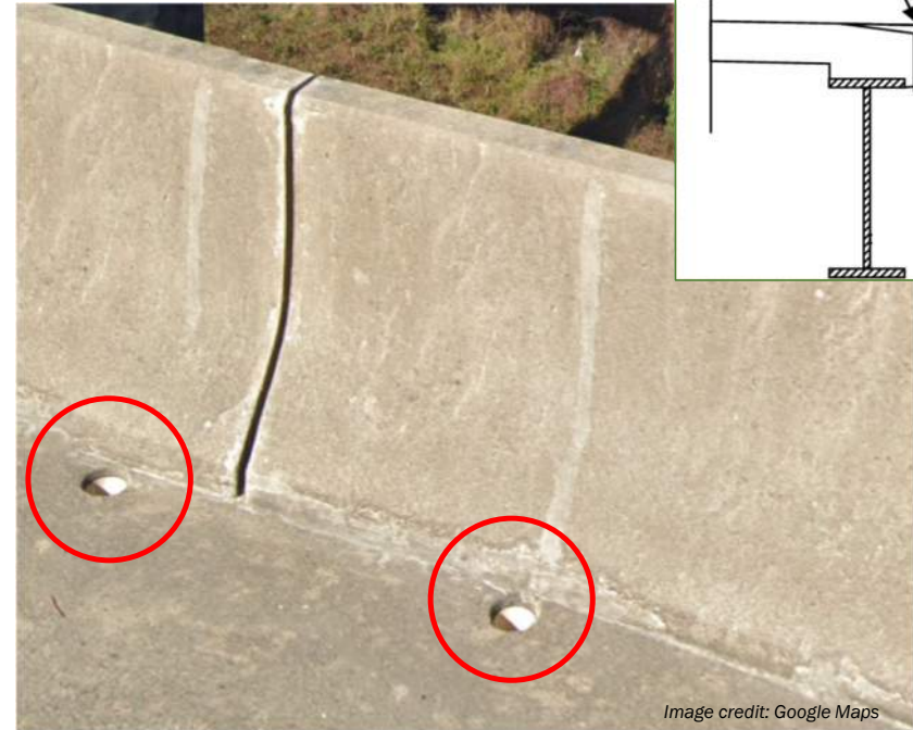
Drainage through the deck only no downspout
