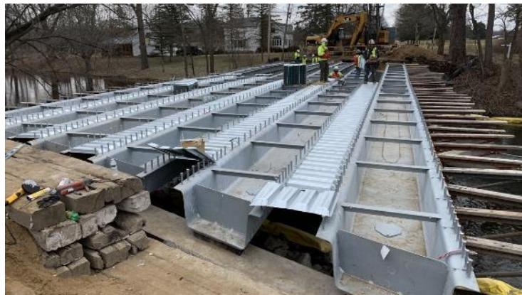
Press-Brake-Formed Tub Girders
