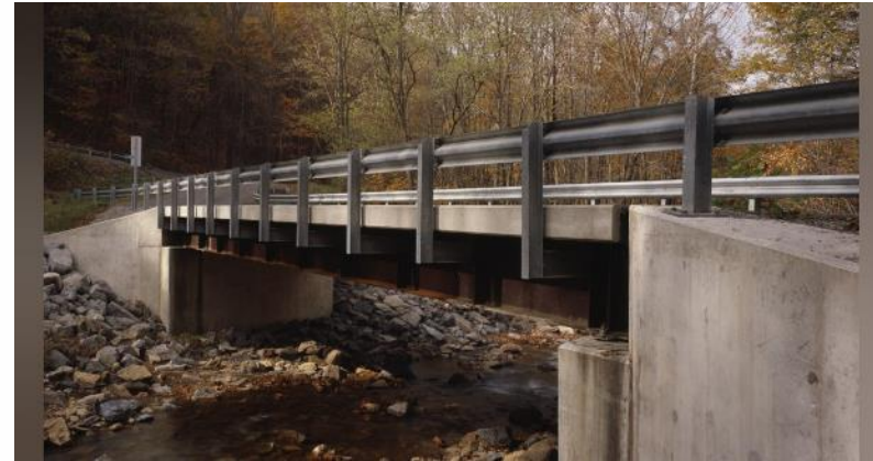
Rolled Beam & Plate Girders
